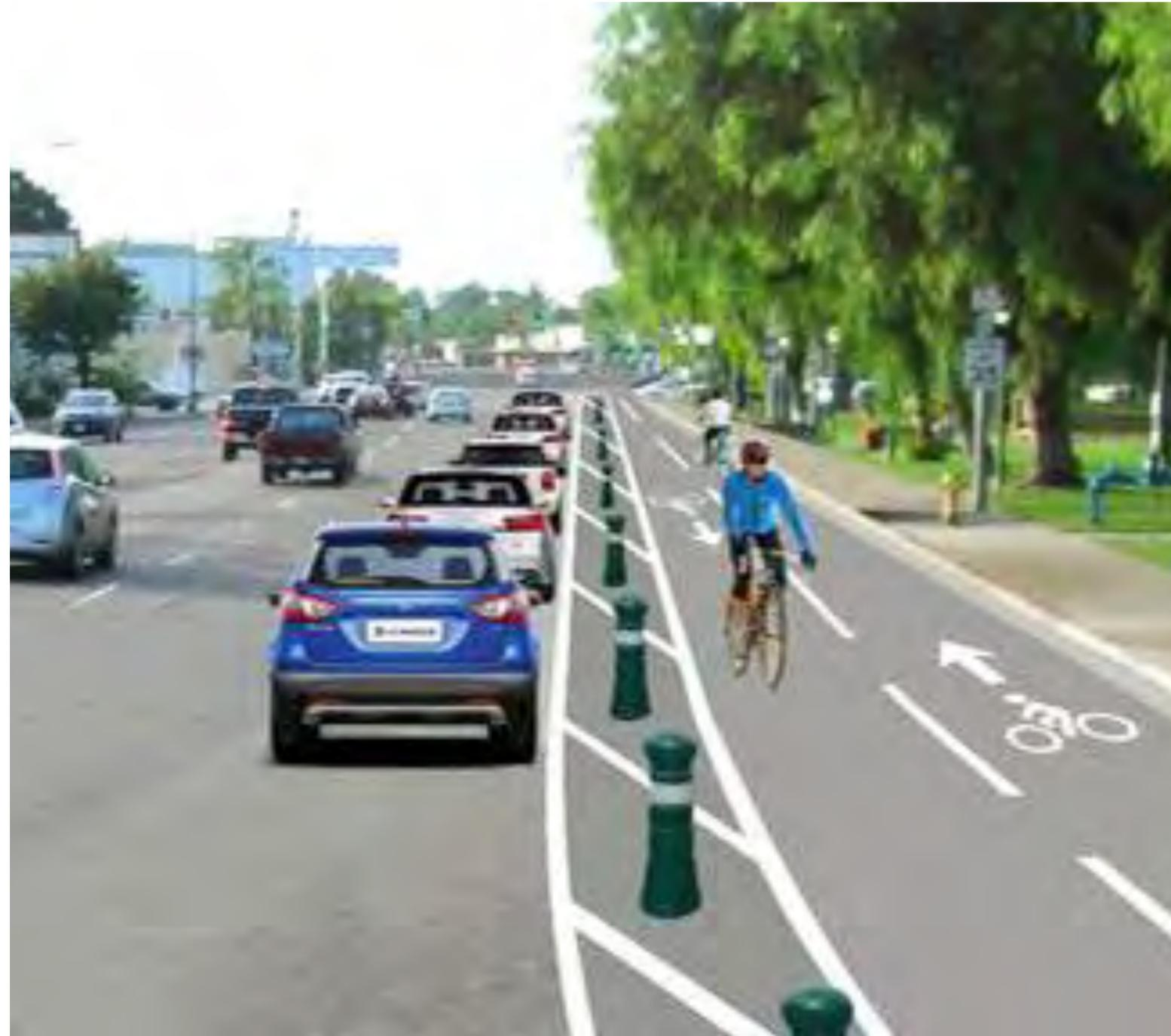
Figure 68. Class IV two-way bollard protected bike lanes
